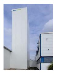
To increase the existing facility capacity, a Kardex Remstar Shuttle XP VLM can be installed outside the building and walled in with pass-through access.
